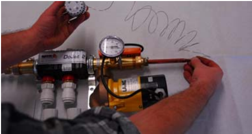
Step 10: Insert sensor in immersion sleeve. DO NOT bend or flex sensor tube!
