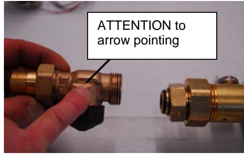
Step 9: Assemble new thermostatic valve orographically
